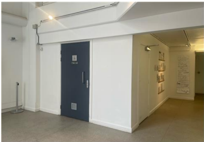
Door to the Accessible toilet from Artspace
