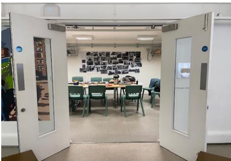
Ground Floor doorway from Artspace to Small Artspace, width 1450 mm
