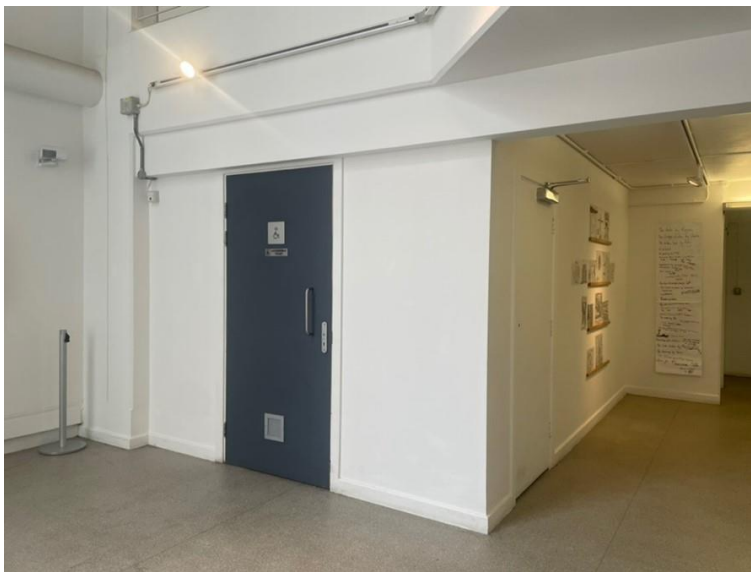
Ground Floor Accessible toilet door from Artspace
