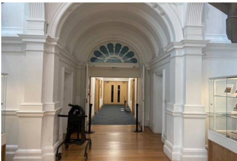
Doorways from entrance hall to Henry Moore Lecture Theatre, widths 1900 mm
