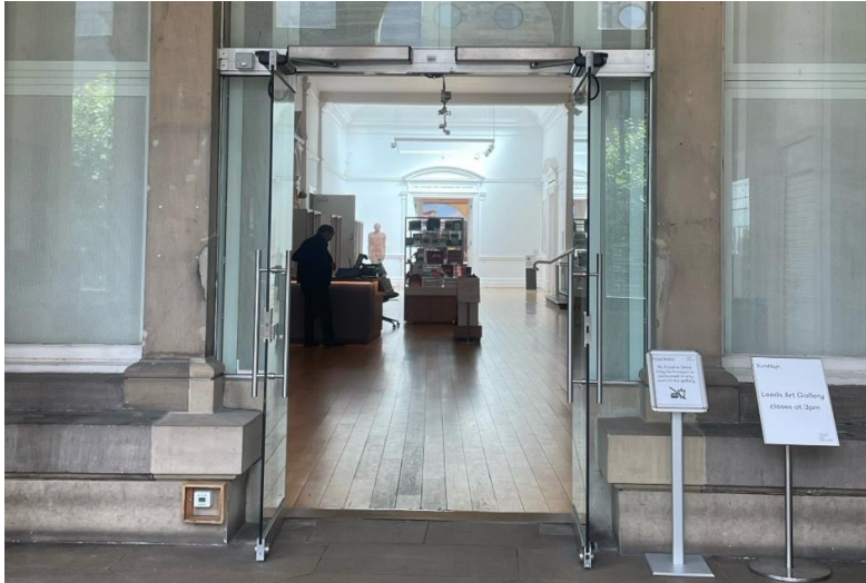
Gallery inner entrance doors
