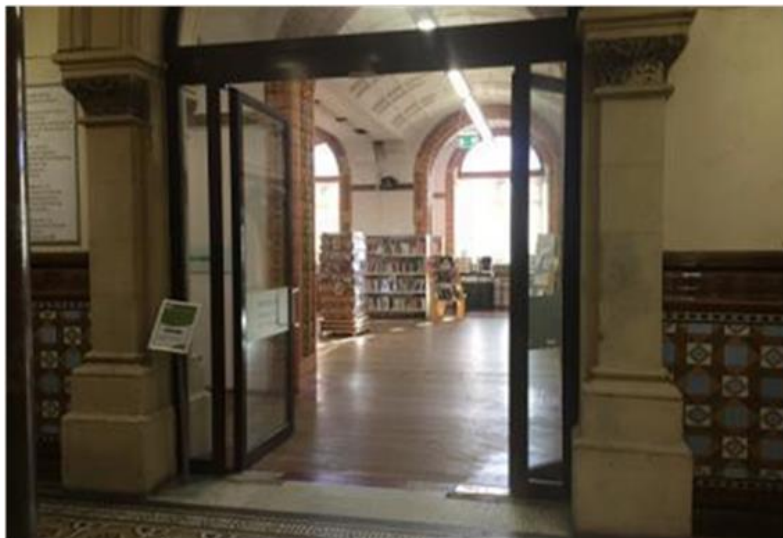
First Floor doorway to the Art Library from lift, width 1630 mm
