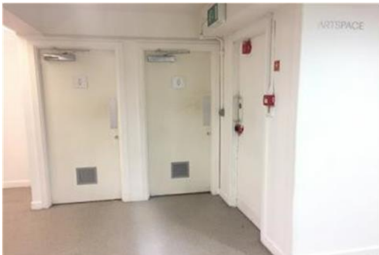
Ground Floor doors to public toilets in Artspace
