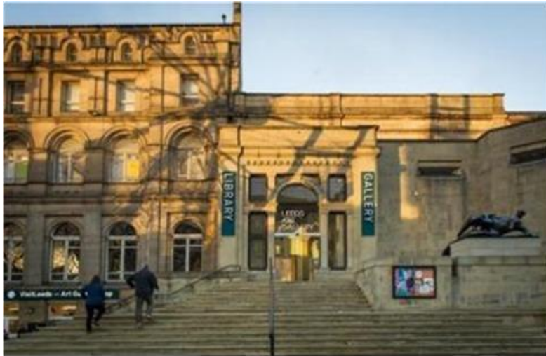
Stairs and gallery entrance doorway
