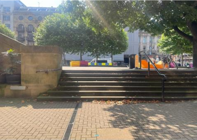
Exterior stairs to Lower Ground Floor exterior level paved area
